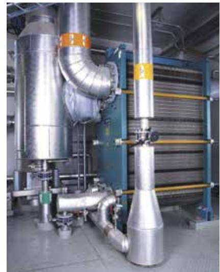
Ethanol condenser at The Absolut Company in Sweden. All the columns at The Absolut Company's Åhus distillery use Alfa Laval reboilers and condensers. The Alfa Laval units were chosen because of their compactness compared to corresponding shell-and-tube solutions.
